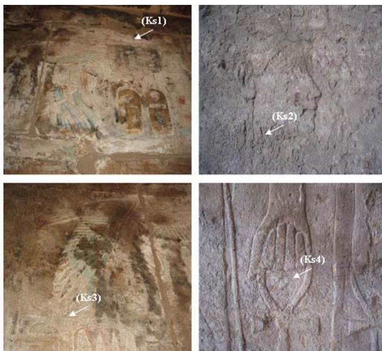
Fig. 1. Crystallization of different salts on the painted surfaces of the festival temple of Thutmosis III, Karnak complex temples. The locations of the collected salt samples are also shown.
